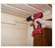
**STEP 23** - Place the upper side bench on the side bench support rail and line up to the upper rear bench. Using 5x70 screws secure the upper side bench to both the wall of the sauna and the upper rear bench from below. Once the bench is securely in place adjust the metal support post by turning the black base of the post clockwise or counterclockwise as necessary to insure a solid placement on the floor.
