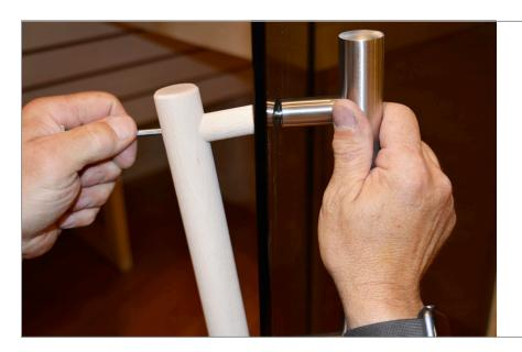
**STEP 32** - Find the door handle and install with the wood portion on the inside of the sauna.
