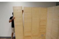
**STEP 7** - Continue the addition of wall elements by adding (3) of the wood wall element sections along the back rail. The wall sections will not screw together, but be sure they are level at the top and firm to each other by tapping in place with a rubber mallet.
