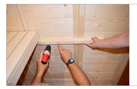
**STEP 21** - Attach the side upper bench support to the side wall by lining up to the rear side bench support. Screw into place with 4x70 screws insuring that the support is level.
