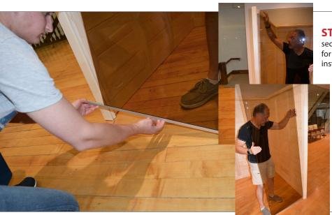
**STEP 15** - Locate the two glass window sections noting that one of them has holes for the door hinges. The instructions show installation with the door opening from left to right, but you can reverse by switching the
