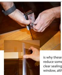
**STEP 31** - Install the hinges onto the glass door and secure to the window. The hinge consists of the hinge bracket, hole spacers, bracket cleat and hex screws. Be sure the screws are snug before mounting the door. NOTE: There is an intentional gap between the bottom of the door and the floor as well as between the glass panels. A sauna must have airflow, which
