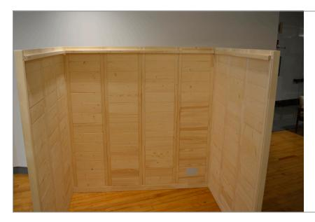
**STEP 14** - The sauna will wood wall sections will now be securely in place and held together by means of the attached roof support rails.
