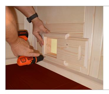
**STEP 29** - Locate the vent cover and position over the wall opening. Attach with (40) 3.5x40 screws.
