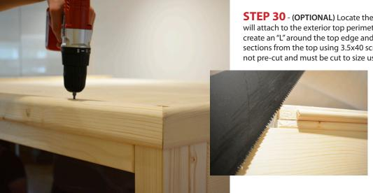
**STEP 30** - (OPTIONAL) Locate the exterior roof trim pieces. These will attach to the exterior top perimeter of the sauna. The pieces create an "L" around the top edge and will be screwed to the roof sections from the top using 3.5x40 screws. NOTE: The trim pieces are not pre-cut and must be cut to size using a hand saw. If the sauna is being placed the corner of the
