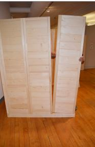
**STEP 10** - Add two more wood wall element sections along the left wall. The wall sections will not screw together, but be sure they are level at the top and firm to each other by tapping in place with a rubber mallet.
