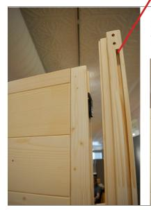
**STEP 6** - Locate one of the 90° corner posts that has clips on one side and a glass groove with 2 holes on the other. Be sure the holes are to the top and facing towards the inside of the sauna. Line up the side with the post with clips to the element section with clips. Raise the post several
