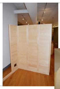
**STEP 5** - Place the next 2 element sections on the right side wall. There will be no screws used in these elements, but be sure the elements are firmly placed to the bottom rail and that the flat top sections are flush to each other. NOTE: THE FRONT ELEMENT SECTION ON THE RIGHT SIDE WILL HAVE 3 CLIPS ALONG ONE EDGE. THESE SHOULD FACE THE FRONT OF THE SAUNA.
