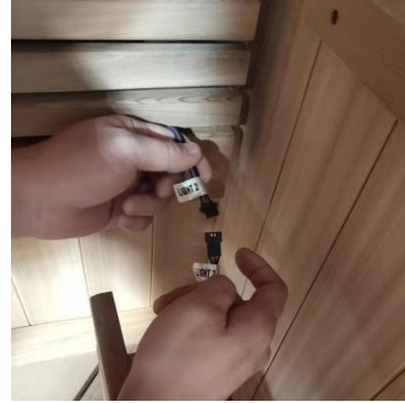
Rear Right – Corner Light Connection
