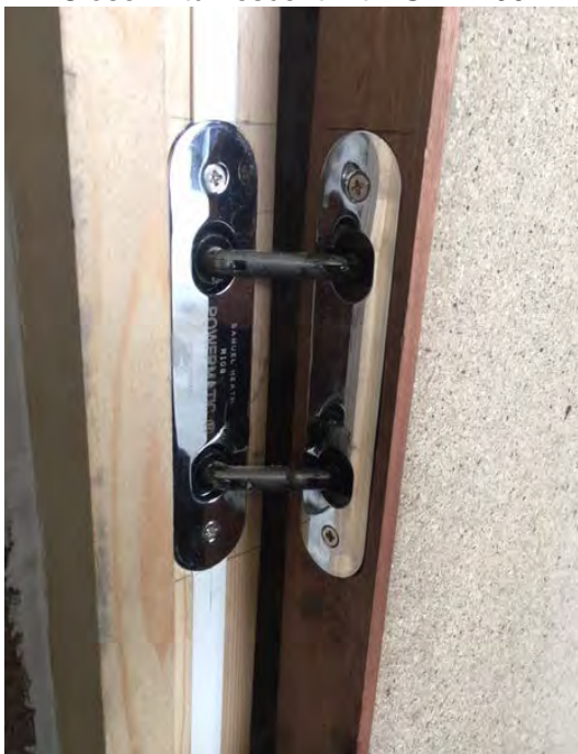
Concealed closer installed – Doorset A
