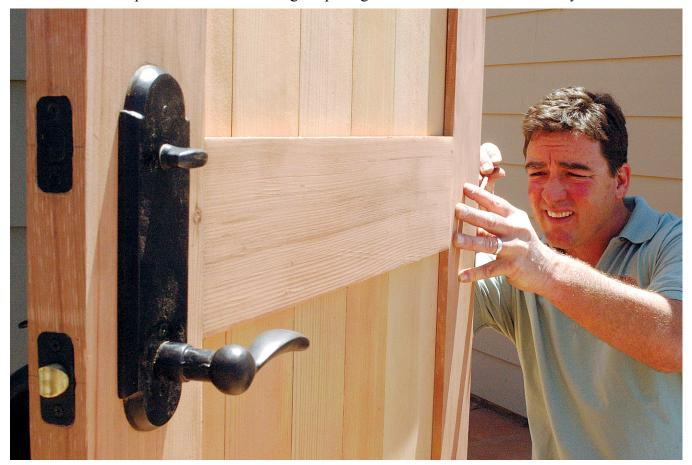
Shannon Williams installs a hinge on a custom gate he designed for Davis and Monica Terrazas. Williams created a gate that would blend with the home's siding. He is looking into installing a self-closing hinge. (Shaminder Dulai/Sentinel)
