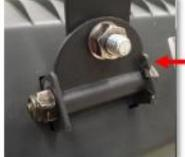
Heater bracket installed outside upper tab.
