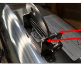
Heater bracket installed between upper and lower tabs.
