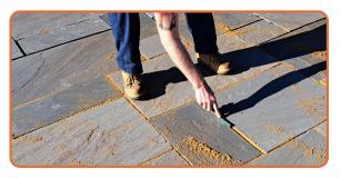
\* Ultimate Joint Compound coverage will vary depending on joint and product type; Wider joints will reduce coverage.
