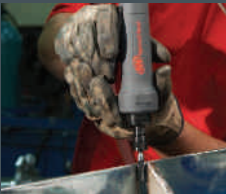
Weld cleaning and smoothing
