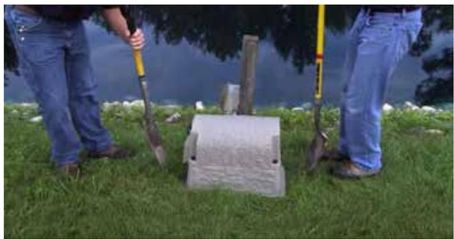
**1.** Place the cabinet on the ground in the selected location and mark an area 6" wider than the base of the cabinet on all sides.
