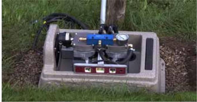
**3.** Place the cabinet onto the stone base, and use your level to make sure the cabinet is sitting secure and level.
