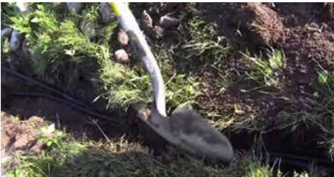
Backfill the airline trench in a few areas to temporarily keep the airline in place until installation is complete.
