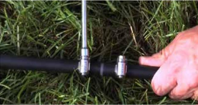
Unroll the EasySet weighted airline and remove any twists. Join enough sections of weighted airline, using 3/8" or 5/8" connector kits, so that the airline can rest on the bottom of the pond, from the pond's edge out to the planned location for each diffuser. For Option B installations, connect the weighted airline to the direct burial airline or Remote Manifold Kit at the pond's edge.
