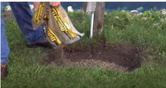
**2.** Move the cabinet and remove the sod from the area, filling in with small stone or gravel. This allows for a firm base for the cabinet and for drainage. Open the aeration cabinet by unscrewing the 4 lobed thumb screws. Gently lift the cabinet lid and lay on its side next to the base.
