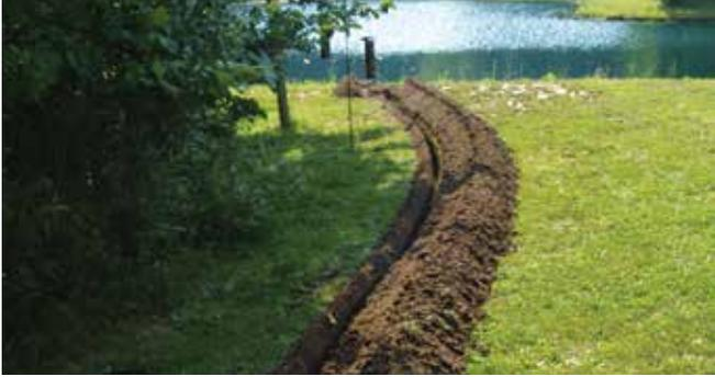
**1.** Using your shovel, dig a trench from the cabinet to the pond's edge. This trench should be a minimum depth of 8" to protect the airline. We recommend having utility lines marked before you begin digging.
