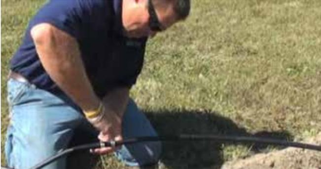
**STEP FOUR: Connect Airline(s) to the Compressor Manifold**
