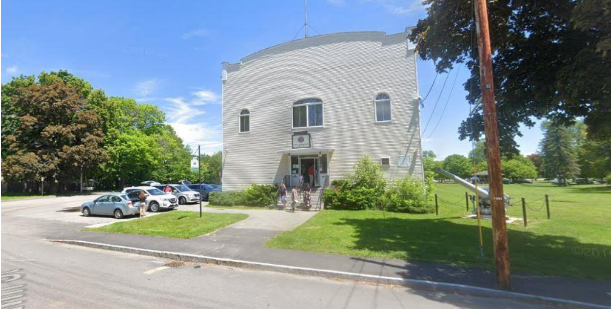
View of Legion Hall and parking area.
