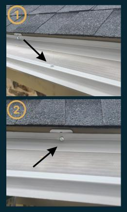
Straight Runs: Work left to right as viewed from the ground. Lay Leaf4go Micromesh completely flat over existing gutters with the front edge of the panel lined up with the top front edge of the gutter and the back edge lying on the drip edge.
