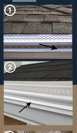
Straight Runs: Work left to right as viewed from the ground. Lay Leaf4go gutter guards completely flat over existing gutters with the front edge of the panel lined up with the top front edge of the gutter and slide the back end under the first shingle.
