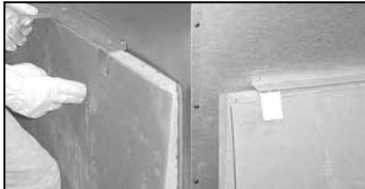
Figure 3.6 Unpacking Back Refractory
