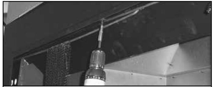
Figure 3.9 Removing the Screen Rods
