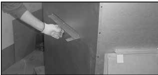
Figure 3.7 Bending Refractory Shipping Tabs Back Down
