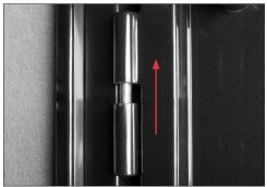
The door must be clear of frame for removal. Lift straight up to avoid damaging bolts.
