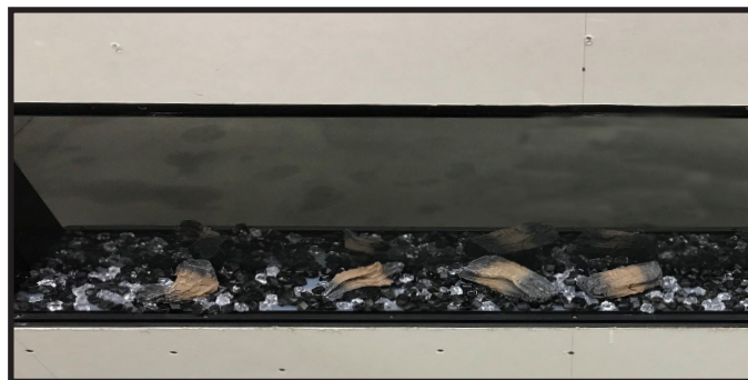
Figure 4.10 Media and Small Logs Installation
