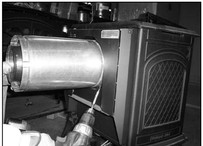
Figure 8 Fasten SLP Vent to Rear Vent
