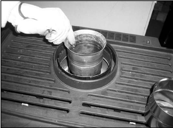
Figure 10 Remove SL-D Adapter
