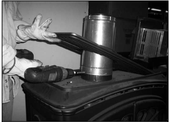
Figure 7 Fasten SLP Vent to Stove
