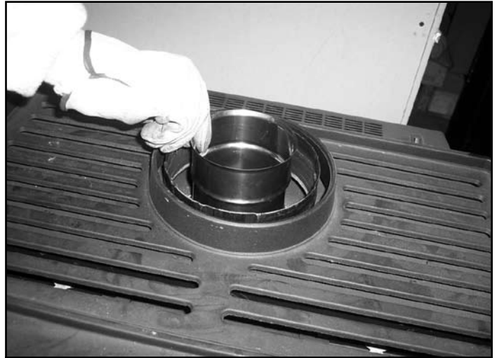
Figure 11 Install SLP-SAM Adapter
