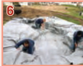
6 Install Liner and Underlayment
