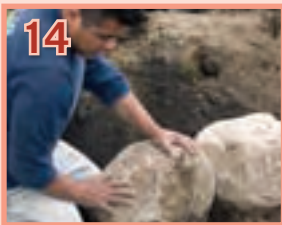
14 Build Retaining Wall
