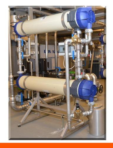
"Bin-X ultra filtration systems reduce the conditions for biological growth, and accordingly also for Legionella, in water systems. The system does not add any chemicals to the water, not even during flushing"
