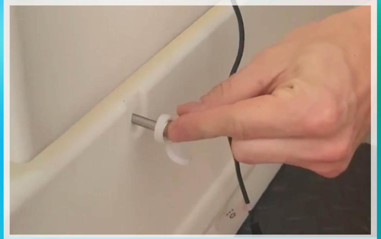
Insert the bolt all the way through the drilled hole.
