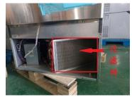
Use a nylon brush to remove dust from the filter;
