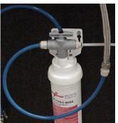
**6.** Connect small flush hose to small fitting and point flush tube into drain pipe.
