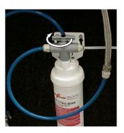
8. Turn arrow on flush valve handle towards the 3/8" inlet to the machine. Check for leaks around filter.
