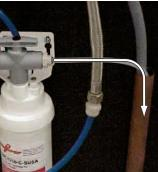
7. Turn arrow on flush valve handle towards the small flush tube (see arrow on top of the valve). Turn on water supply and flush for about 1 minute.
