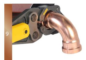
Place the adaptor jaw over the pins on the collar, check that the fitting is still matching up to the insertion depth mark on the tube. Press the trigger on the tool and hold down until piston retracts.
