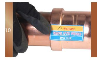
Remove the adaptor jaw from the collar, then the collar from the fitting. Now you can remove the sticker from the fitting to confirm press is complete.
