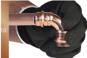
Inspect fitting to ensure press is complete.
