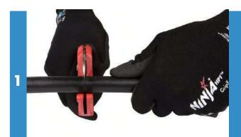
With a set of pipe cutters /shears cut the pipe at 90° ensuring the pipe is square on the end.
