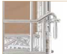
Protective cover on exposed wire ends.
