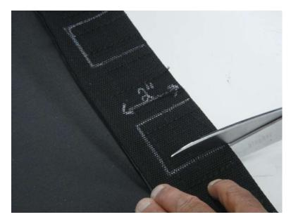
Figure 14.1 - Cut out Velcro Tab Binding at each Clamp Location
