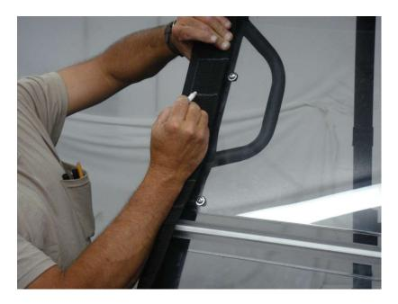
Cut the webbing strip with household scissors. **AGAIN, DO NOT CUT INTO THE BINDING.** Seal the frayed edges with a lighter. Have a wet cloth handy to dab the edges if needed.
