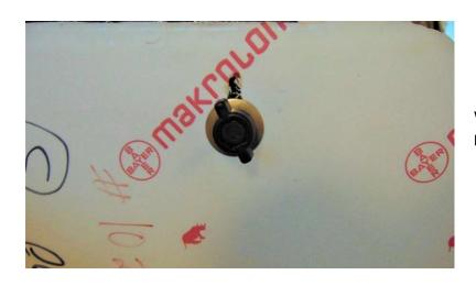
Wingnut and neoprene washer should be positioned on the outside of the back panel.
