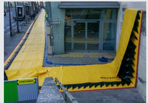
Lifting & securing the ends, helps seal the edge against water infiltration
