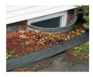
Flood Barriers can be left in place for about a season to assist in redirecting water or can be disposed of in the garbage
