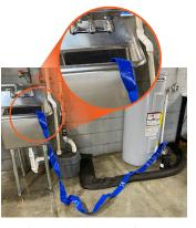
Run hose to an area where water can run off and will not cause additional water issues
