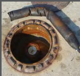
Remove saturated sock & replace if necessary
