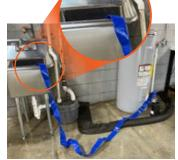
Run hose to an area where water can run off and will not cause additional water issues
