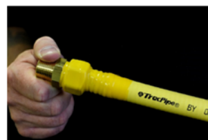
The tape should then be wrapped back over the first layer, over the fitting nut and up to the edge of the shoulder of the fitting
