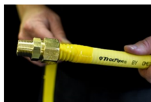
With the tape stretched very tightly wrap onto the outer cover
