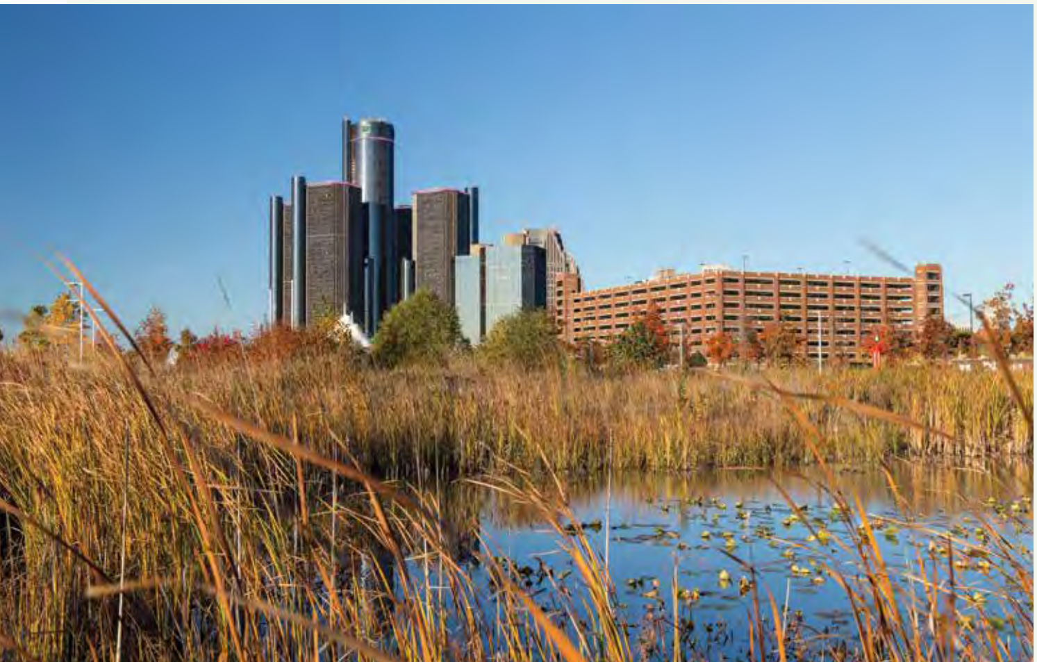
Green Stormwater Infrastructure. Detroit, MI. © Michael David-Lorne Jordan
