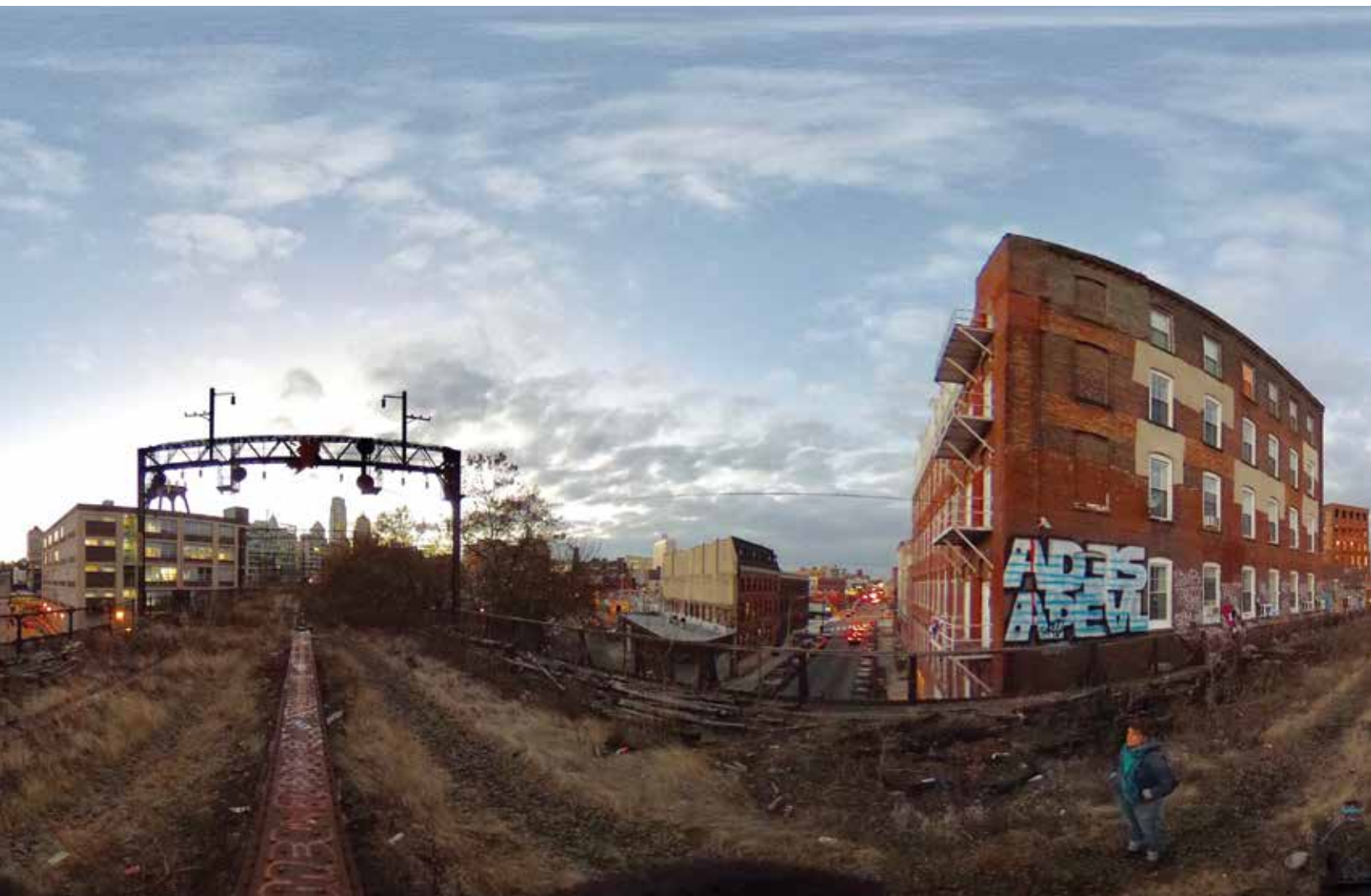
Reading Viaduct. Philadelphia, PA. © Marc Steiner
