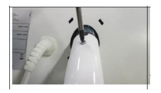
Once the pole is back in place you will need to replace the screw with the philips head screw driver. Once the screw is tightened then move the plastic cover that is outside the frame of this picture back up the pole and into the slots.
