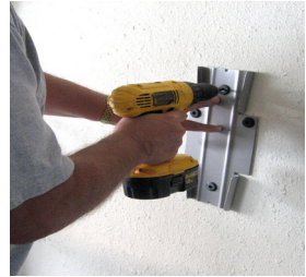
Fig. 2 Mount the wall bracket.
