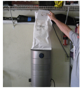
Fig. 1 You will need to be able to remove the bag from the top of the unit. Be sure to leave enough room when mounting.
