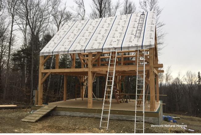
**INTELLO X** can be used as a temporary roof during the construction phase for roof pitches of 3:12" (>15°) and higher walkable and waterproof
