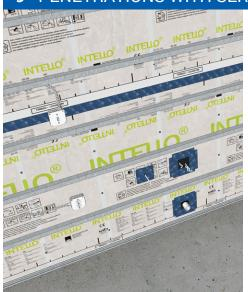
Airseal pipes and cables with ROFLEX and KAFLEX air sealing sleeves. The cable sleeves and ROFLEX 20 are self-adhering with integrated TESCON VANA patches. Other ROFLEX pipe sleeves are adhered to INTELLO with TESCON VANA.
