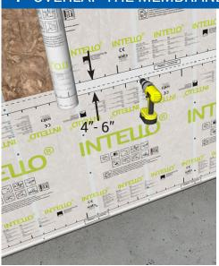
Using the printed markings as a guide, overlap the next row of INTELLO over the bottom sheet and fasten along the bottom edge. As in Step 3 - pull the membrane up into a taut triangle and fasten at the upper edge.
