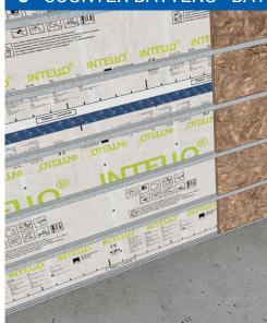
Optional: add horizontal counter battens spaced max. 20" apart to form a service cavity in which wiring and services can be placed. Cavity can also be insulated before the sheetrock is installed.
