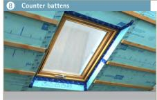
Add horizontal counter battens spaced max. 20" apart before the dense packed insulatio is blown in
