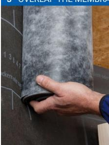
After the first layer is applied begin the second row. Use the printed markings as a guide and shiplap the WRB by 6" (150 mm).
