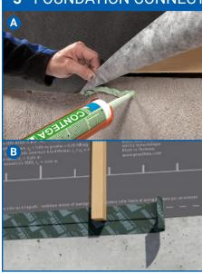
A. Use CONTEGA HF to connect to concrete foundation, or other rough surfaces. Make sure substrate is stable or use TESCON PRIMER RP. Apply a 1/4" (6mm) wide bead (wider on rough surfaces). Press the membrane into bead, with room for expansion/contraction of structure. Do not press adhesive completely flat. Let cure for 48 hrs.
