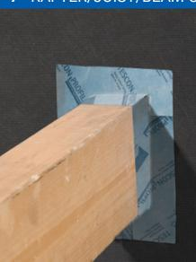
Waterproof and air sealed connections to beams, can be made with TESCON PROFIL tape. Cut the tape 2" (50 mm) longer then the beam dimensions.
