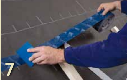
Taping roof underlay
