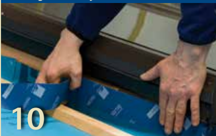
Sealing external junctions
