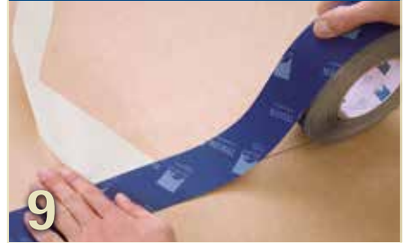
Sealing sarking boards
