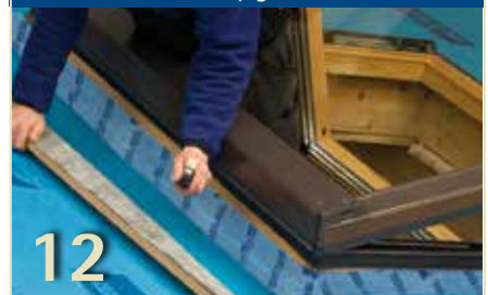
Details for underlay gutters
