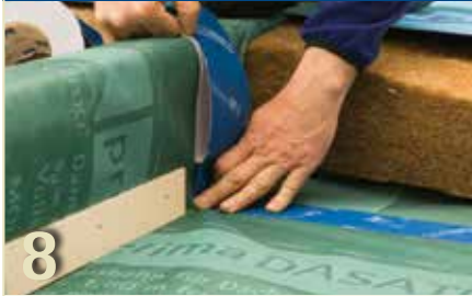
Taping Sub-and-Top membrane
