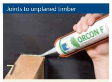
Use CONTEGA OR-F joint adhesive on unplaned or roof beams, applying a continuous bead approx. 1/4" (5 mm) thick (more may be needed on rough sunstrates).
