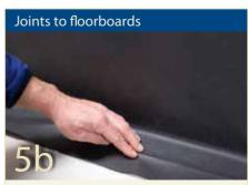
Lay the membrane on the adhesive bed, leaving an expansion joint and do not press the glue down completely to allow for differential movement at the joint.
