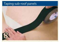
Use TESCON INVIS for joints on sub-roofs made from wood (MDF), positioning the tape centrally over the joint, unrolling and sticking down over the joint piece by piece then pressing firmly to secure the tape. Prime softwood fibre panels with TESCON PRIMER RP.
