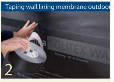
For invisible taped joints on and joints between wall lining membrane (e.g. SOLITEX WA) behind back ventilated façades, position TESCON INVIS centrally over the overlap, unroll and stick down over the joint piece by piece.
