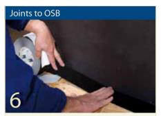
To create windproof joints between wall membrane and smooth, non-mineral surfaces such as woodbased panels or planed wood, place TESCON INVIS centrally over the joint, unroll and stick down over the joint piece by piece.
