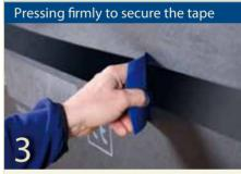
Press firmly to secure the tape, ensuring there is sufficient back-pressure, for example using a pro clima PRESSFIX to do the job effectively and to protect your hands.
