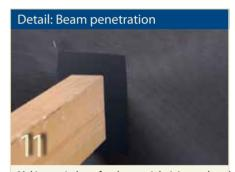
Making a windproof and water tight joint to planed rafters or roof beams with TESCON INVIS. Bonding sequence: 1st bottom, 2nd left and right hand sides, 3rd top. Use ORCON F joint adhesive to bond joints to unplaned rafters or roof beams.
