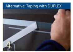
Alternatively, you can use DUPLEX double-sided tape to tape over the overlap. Lift the top layer of membrane, apply the DUPLEX on one side, pull the release paper off piece by piece and stick down, ensuring there is sufficient back-pressure, and press hard
