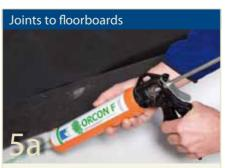
To bond joints on floorboards, masonry or concrete or other rough substrates, use CONTEGA OR-F joint adhesive. Clean the substrate and apply a continuous bead approx. 1/4" (5 mm) thick (more may be needed on uneven substrates).
