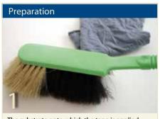
The substrate onto which the tape is applied should be load bearing and stable, dry, smooth and free from dust, silicon and grease. Brush down all surfaces and vacuum clean or wipe with a cloth if necessary.
