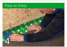
Firmly press tape onto wall and floor. The pressing aid pro clima PRESSFIX is particularly efficient and protects your hands.
