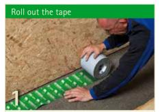
Roll out the tape to the required length and cut to size.
