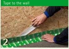
Fold the tape at an angle and push into the corner of the wall/floor. Piece by piece, remove the first release paper and gradually stick tape to the wall.
