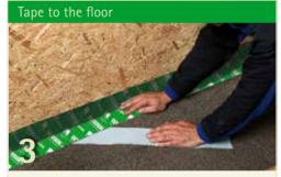
Piece by piece, remove the second release paper and gradually stick tape to the floor.
