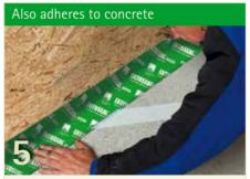
EXTOSEAL FINOC can also be stuck directly onto concrete. Where necessary, prepare the subgrade with TESCON PRIMER RP.
