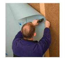
DB+ can be unrolled and stapled either downwards or across the rafters. Lengthwise fitting is shown here. As rolls are available in various widths, there is usually very little waste.
