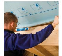
For sawed beams or rafters, apply the joint adhesive ECO COLL in an approximately 5 mm thick adhesive bead. With rough surfaces, increase the bead size as necessary.
