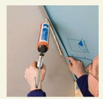
For joints to plastered gable walls apply the natural latex adhesive ECO COLL directly from the cartridge in an approximately 5 mm thick adhesive bead. With rough surfaces, increase the bead size as necessary.
