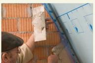
If the wall is subsequently plastered, then CONTEGA PV need only be embedded in the middle layer of the plaster. To do this, push back the fleece and reinforcement, apply plaster to the wall behind CONTEGA PV. lav the fleece and reinforcement in the fresh layer of plaster and then complete the plaster work. Finished.
