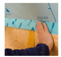
Just as important as the sealing of overlaps are joints to adjacent structural components. UNI TAPE is used for joints to smooth, non-mineral structural components (such as the jamb wall made of OSB panels shown here). Gable walls are treated analogously.
