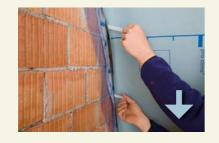
Apply the vapour barrier. Remove the strips of release paper from the back of the CONTEGA PV and affix the fleece to the air-proofing layer using adhesive tape. Press firmly to
