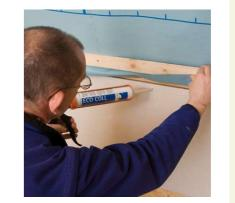
The joint adhesive ECO COLL is applied to adjacent mineral structural components or rough wooden components (e.g. plastered walls or sawed rafters) directly from the cartridge in an approx. 5 mm thick adhesive bead. With rough surfaces, increase the bead size as necessary. Lay the vapour check, with an expansion joint, in the adhesive bed. To allow for movement of the parts, do not press the glue completely flat. Pressure laths are usually not required on stable surfaces.
