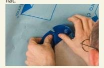
Seal the corners with short pieces of TESCON No.1. In the centre of the adhesive tape, cut halfway through. Then it is easy to shape.
