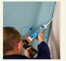
For connections to insulated, doublelayer chimneys, apply approx. 3 cm of DB+ to the chimney. Apply an approx. 5 mm thick adhesive bead (more if necessary) with ECO COLL and lay the membrane, with an expansion joint, in the adhesive bed. Do not press the adhesive completely
