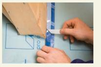
In the second step, simply remove the rest of the release paper and finish sealing.
