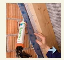
Defined plaster joint with CONTEGA PV. Affix the fleece at intervals and as far as possible in the corner using ORCON F.
