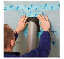
If pipes or cables go through the air-proofing layer, they too must be securely sealed. The most suitable means of doing this is with airproofing sleeves made of EPDM. This flexible material allows a tight fit, and is available in all common diameters. Cable sleeve are selfadhesive. Remove the release paper, push over the cable and stick on. Pipe sleeves are affixed using UNI TAPE. Press firmly to secure the adhesive tape.
