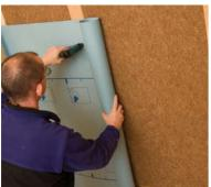
On the interior side, beneath the insulation the pro clima DB+ vapour check and air-proofing membrane is now laid. It protects the thermal insulation from moisture and mould. The membrane has no front and back side and can be fitted with either the printed or the unprinted side facing the room. Staples should be 10 mm wide and 8 mm long and set at a max. distance of 10-15 cm.
