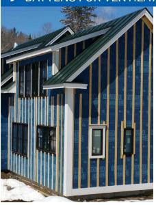
It's recommended to use a vented rainscreen for optimum performance and drying capacity of all Pro Clima WRBs. When constructing a rainscreen a min. 3/4" (20 mm) ventilated cavity is recommended.
