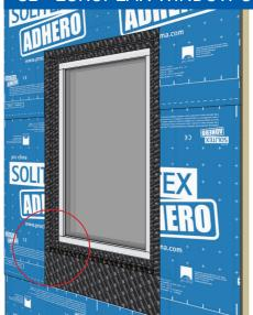
Seal frames with CONTEGA SOLIDO EXO to taped window bucks. Start on the bottom and work your way up for proper shiplapping. Use pre-made L-shaped corners for most accurate sealing of corners. Apply tapes to windows as per manufacturers recommendations and installation instructionsnote drainage planes, condensation weeps etc. Pressurize tape firmly with a PRESSFIX
