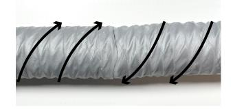
Twist one end of a duct into another, in the direction of airflow. Make sure they overlap at least 2".
