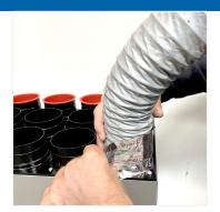
Overlap the end of the flex duct onto the collar of the manifold.
