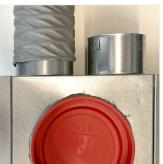
Slide the flex duct halfway over metal collar of the diffuser box.
