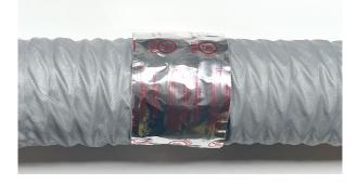
Tape the seam of the overlapping ducts with UL listed tape to secure this connection and ensure an airtight seal
