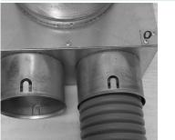
Insert the end of the duct into the collar of the register box. Bend the tabs of the collar carefully so the duct secured - but not punctured. Use soap or silicone spray if necessary
