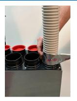
Insert the end of the duct into the collar of the manifold. No o-ring necessary.
