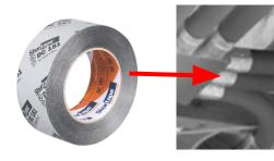
Clean the outside of sleeve and duct. Tape the duct to collar to create a secure airtight connection.
