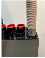
Seal the collar to duct pipe with tape to create a secure airtight connection.
