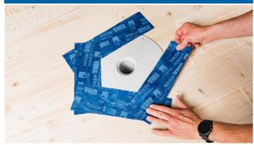
Install a temporary floor drain system that prevents the build up of standing water or have other means to remove pooling water from the membrane (sweeping, mopping etc). The short-term accumulation height should not exceed 1 3/16" (30 mm). Standing water should be removed within 24 hours. Do not leave the membrane permanently wet/submerged.
