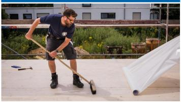
Press the membrane firmly into place using a PRESSFIX XL application tool, broom, or roller.
