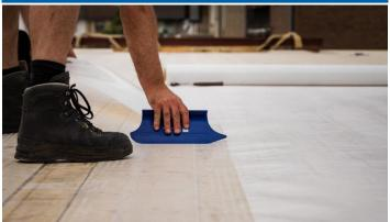
Remove the 10" (250mm) adhesive strip. Pressure apply the membrane firmly into place using the PRESSFIX XL application tool, broom, or roller.
