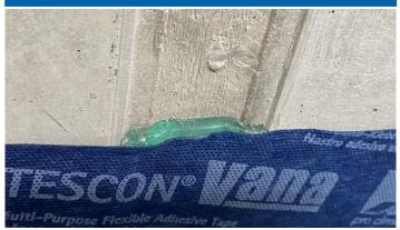
Any gaps or defects are to be covered with TESCON VANA in a waterproof manner or, filled with CONTEGA HF.
