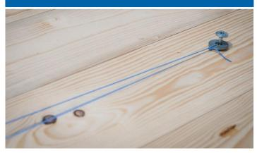
Mark a line on the CLT to position the first ADHERO VISTO edge to be applied.
