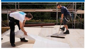
Remove the remaining release paper. Press the membrane firmly into place using a PRESSFIX XL application tool, broom, or roller.
