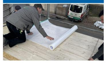
Roll out the membrane along the guideline and gradually adhere it to the substrate.
