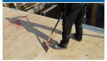
Clean dirt, debris and remove any protruding elements (splinters, nails, screws, etc) that can damage the membrane during installation.
