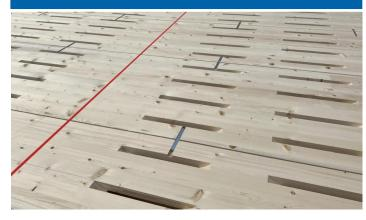
Align ADHERO VISTO with the marking. Plan the installation such that there is continuous adhesion with a flat surface.
