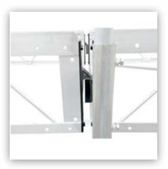
Once the supported section of dock is in the desired position, bring the second, un-supported section into position and align the hooks (male) over the loops (female). Drop the hooks into the loops.
