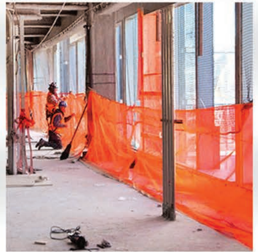
SAFETY DEBRIS NETTING
