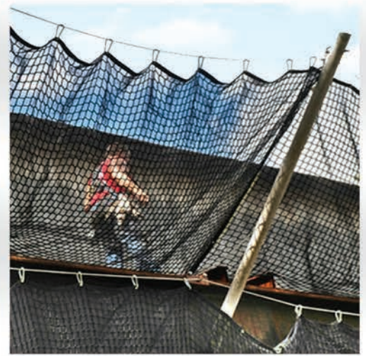
FALL PROTECTION SAFETY NETS
